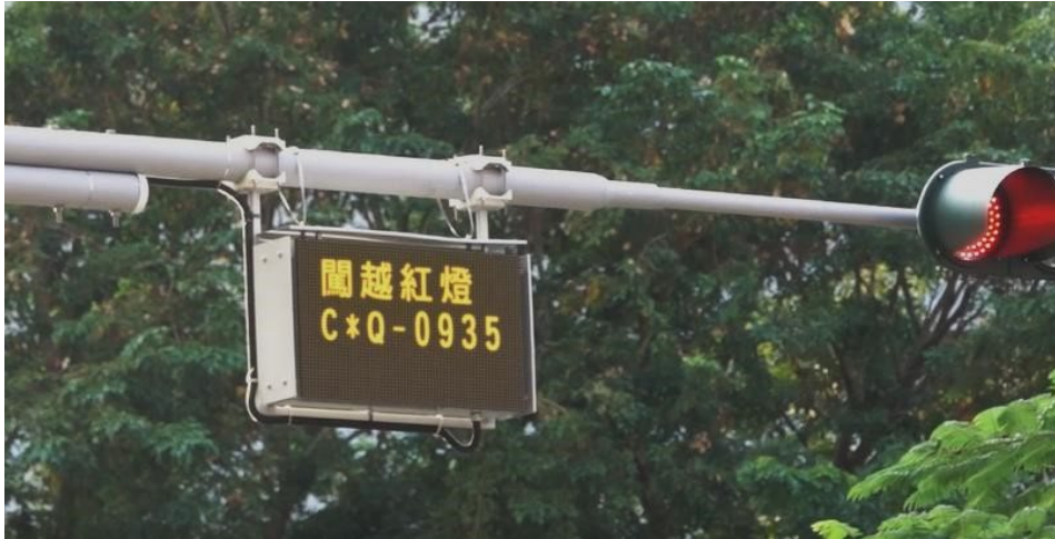
Figure 7 – CMS Digital Signs produced real-time warnings to violating motorists
